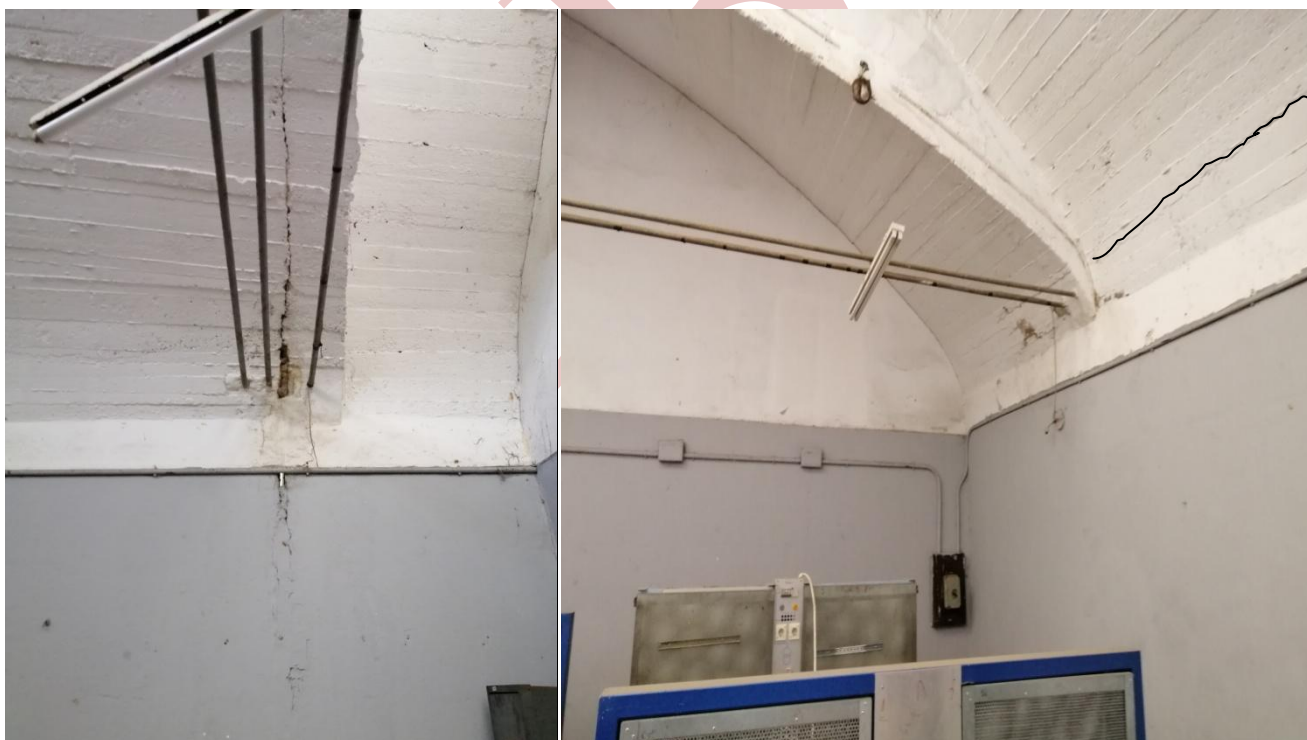
Figure 59 : Apparition des fissurations.
